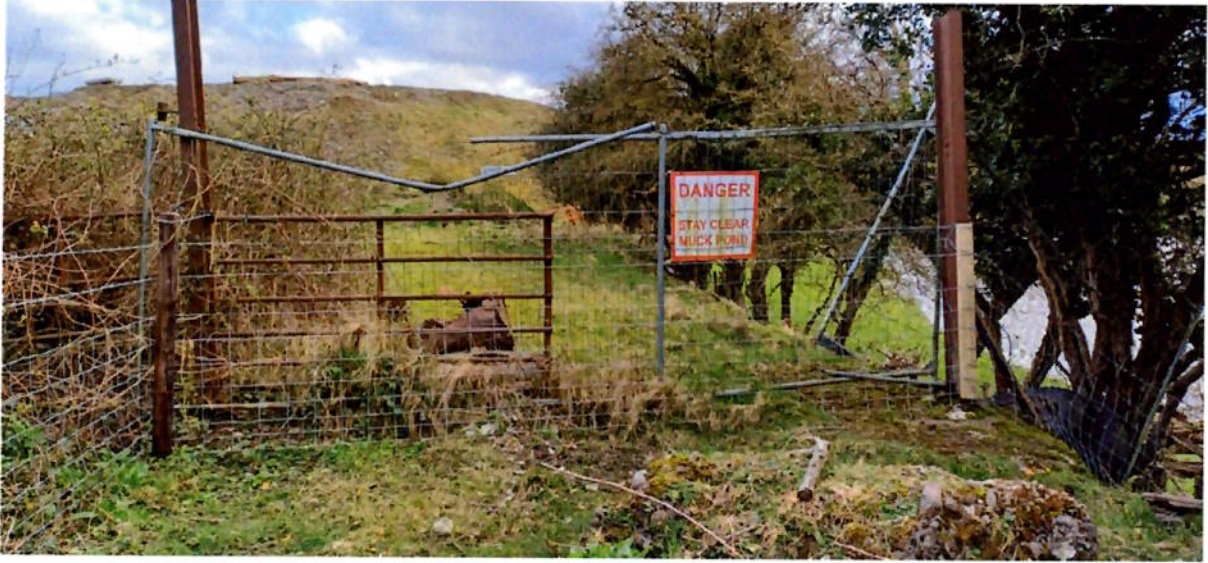
Another access point that does not meet the conditions set down in the planning conditions.
