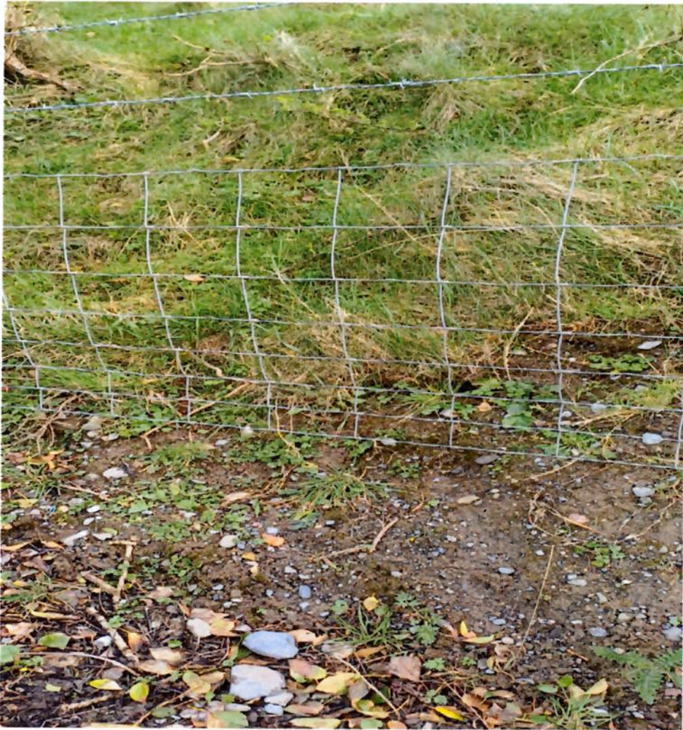
Huge gaps in the fencing at ground level to let livestock or children through.
